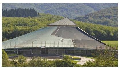
rent that the black part on the right half of the roof constitutes a gigantic patch of over 400 square metres on the wound. The protective waterproof sheathing placed on the roof served to secure the building and prevent rain from flooding the building. The numerous downpours that followed stressed the protection, so much so that seepage into the church occurred in some places.
